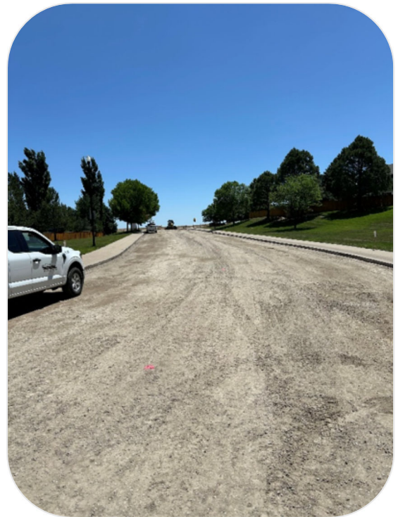
After Mallard Drive Subgrade Repairs
