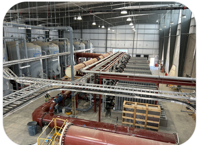
Water Treatment Building Progress
