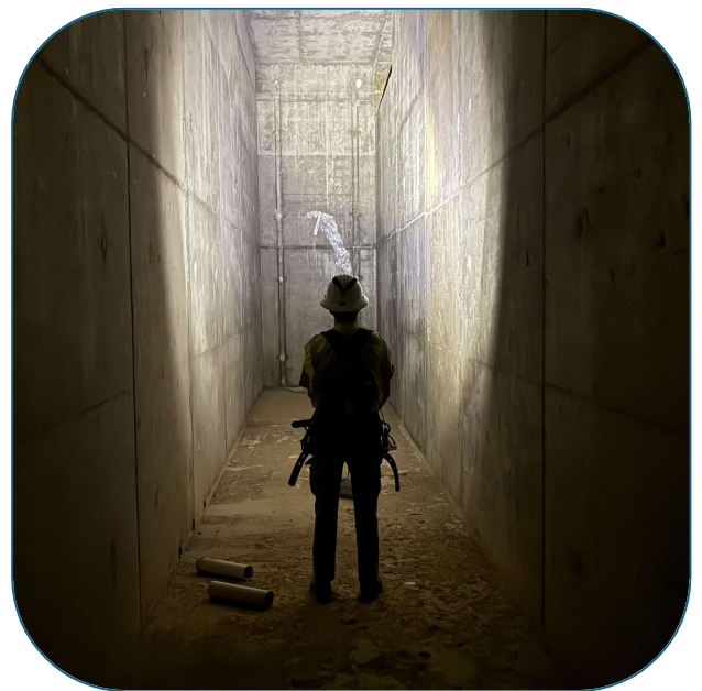
Chief Plant Operator Blayne Banghart Inspection of the New Water Basin Chamber
