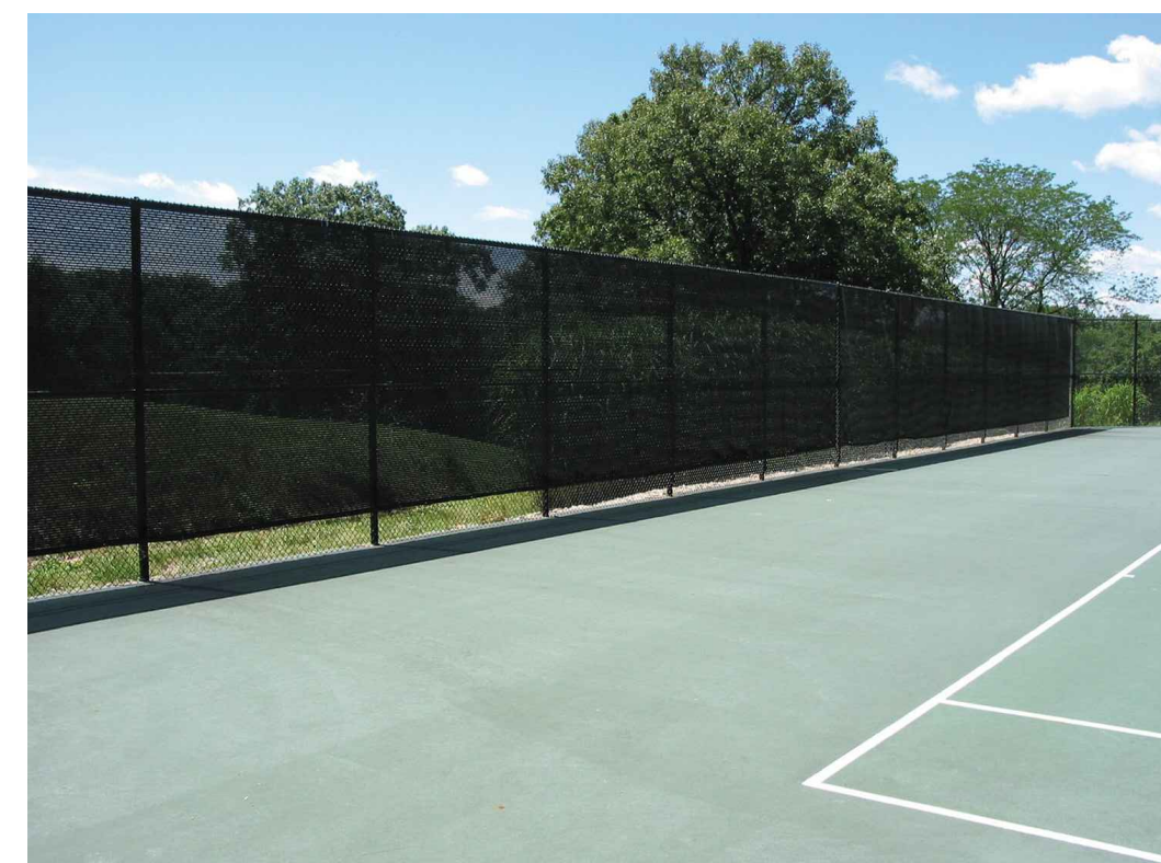
C MULTI-SPORT FENCE AND CLOSED MESH WIND SCREEN MANUFACTURER: NATIONAL SPORTS PRODUCTS; PRODUCT: DOUGLAS POLYPRO PLUS PREMIUM OR EQUAL; MODEL # 21650Z
