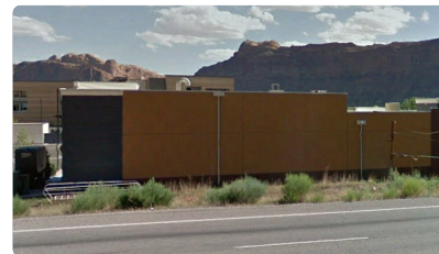
Colorado River Resort WTP
