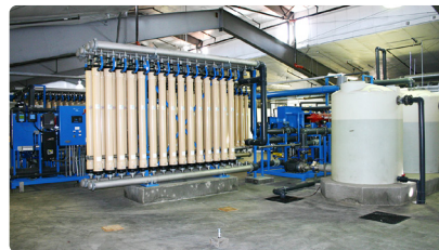
MRW Signal Hill WTP
