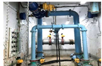
Figure 2-3. Existing Filter Gallery
