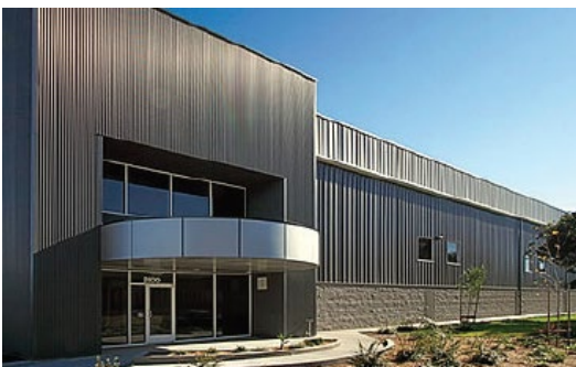
Figure 2-23 Acceptable Metal Panel
