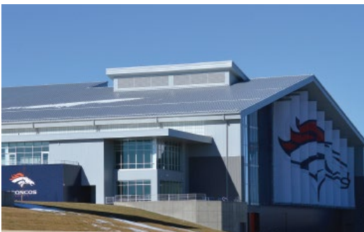
Figure 2-19 Acceptable Metal Panel
