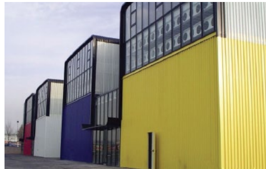
Figure 2-32 Acceptable Metal Panel
