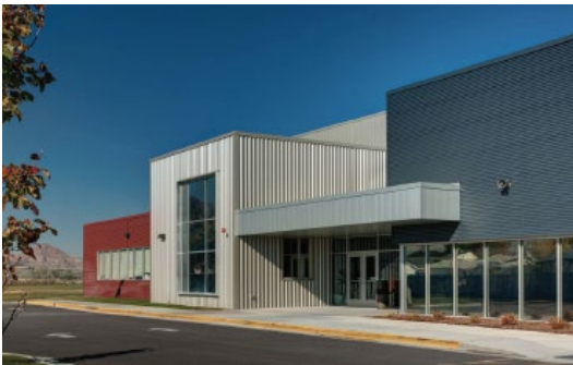
Figure 2-27 Acceptable Metal Panel
