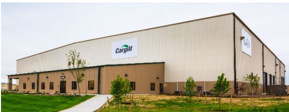
Figure 2-37 Unacceptable Metal Panel
