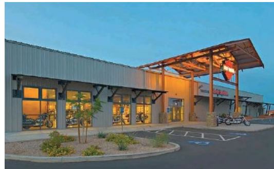
Figure 2-22 Acceptable Metal Panel
