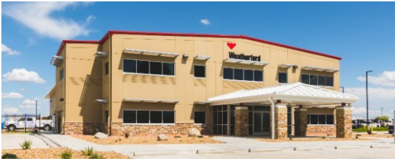
Figure 2-35 Unacceptable Metal Panel
