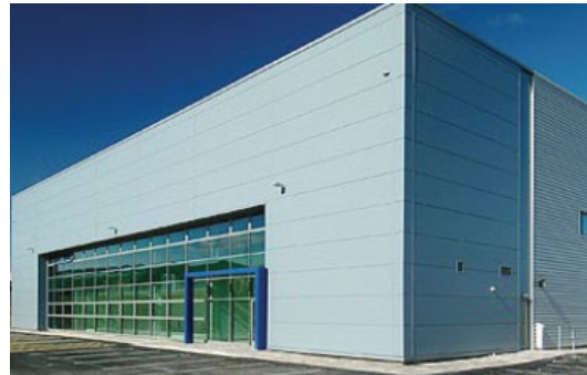
Figure 2-30 Acceptable Metal Panel
