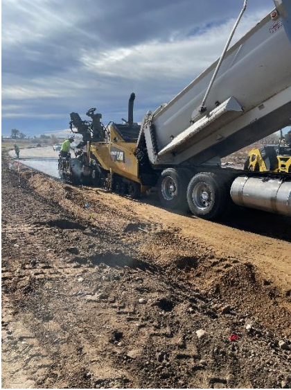
CR3 bottom mat paving
