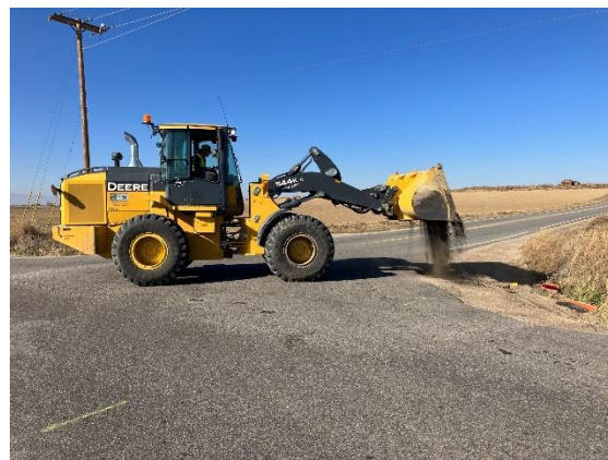
Crews filling corner of CR 50/CR13
