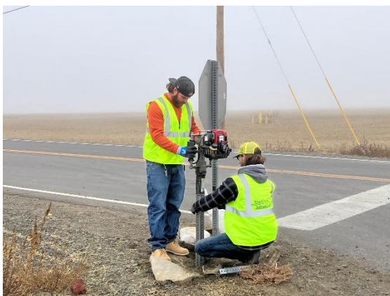
Crews replacing stop sign
