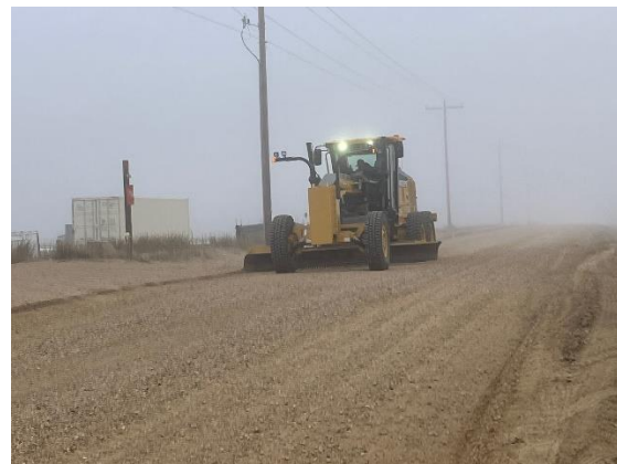
Crews grading CR 42
