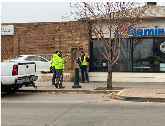
Crews installing Holiday lights
