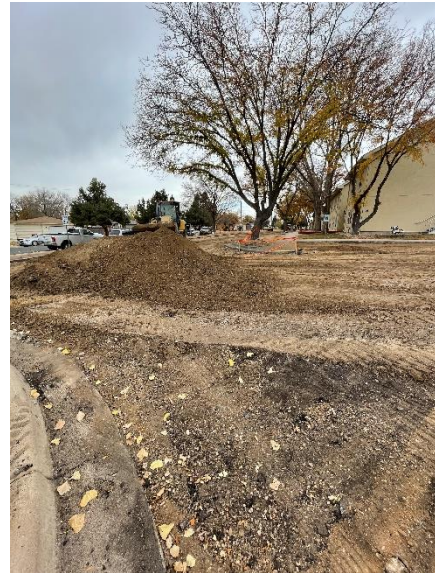
Housing Authority parking lot subgrade work
