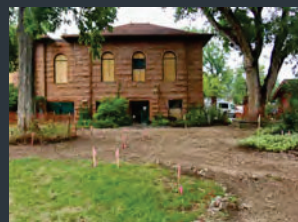
Before and after of the exterior. During demolition, the project team carefully removed the original windows and sent the windows offsite. The glass was restored and reused in the finished project.
