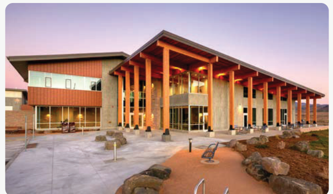
Northern Water - Building A Addition & Renovation
