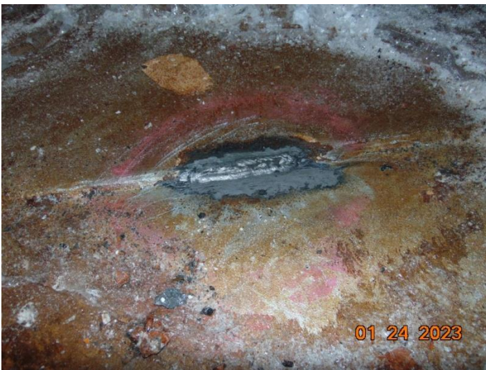
Interior Coating / Floor
