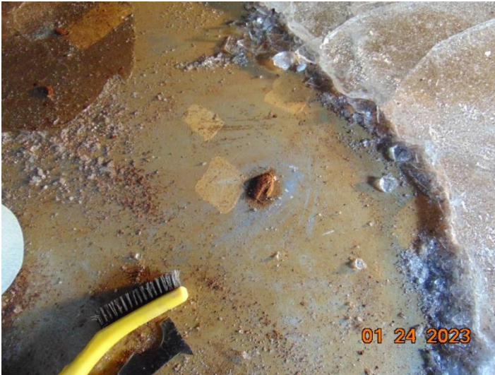
Interior Coating / Floor
