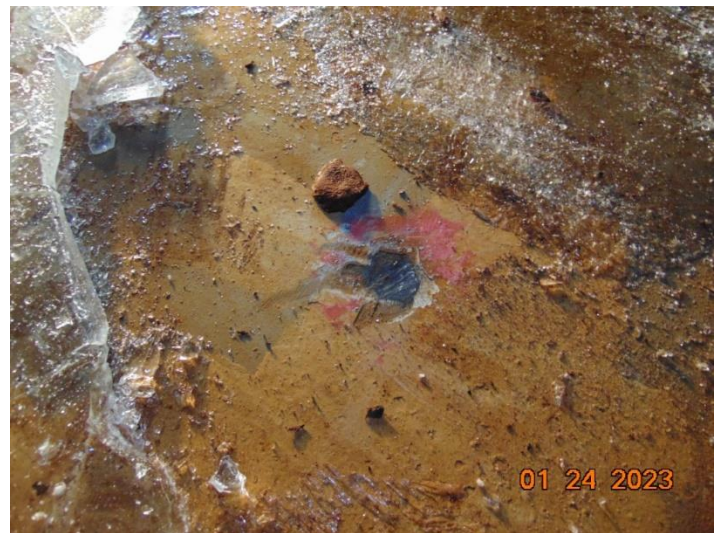
Interior Coating / Floor
