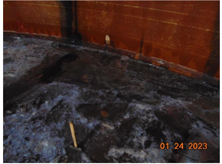
Floor / Shell Connection
