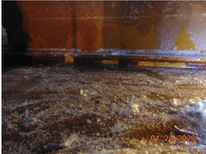
Floor / Shell Connection
