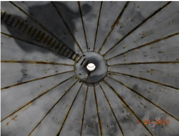
Roof Interior from Floor
