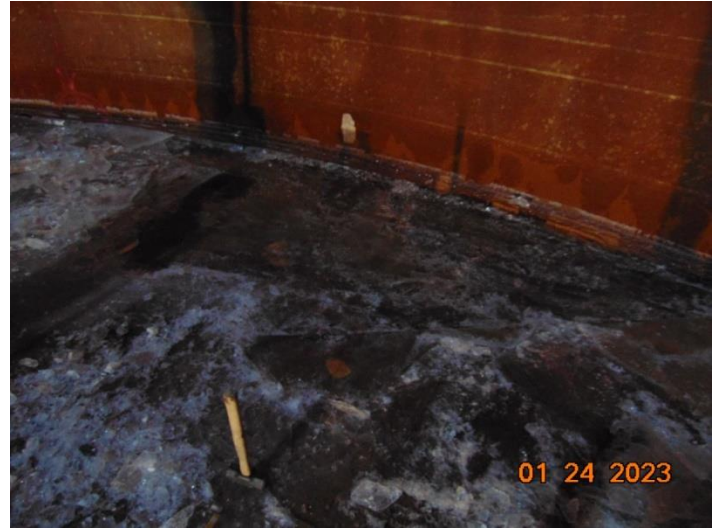
Floor / Shell Connection
