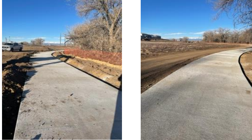
Little Thompson Trail Construction
