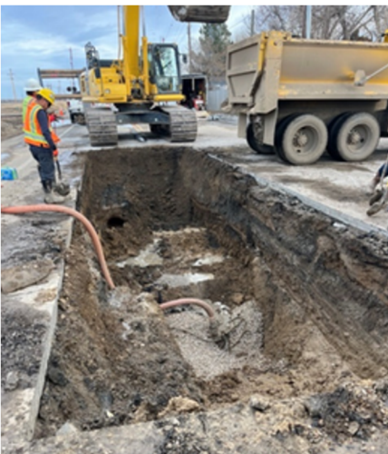
*SH60 Waterline Replacement
