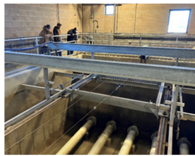
*DAF system maintenance
