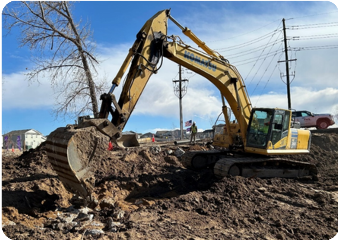
* Construction of Little Thompson River Pedestrian Bridge
