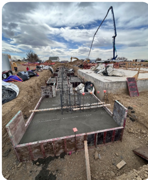
* New Treatment Building
