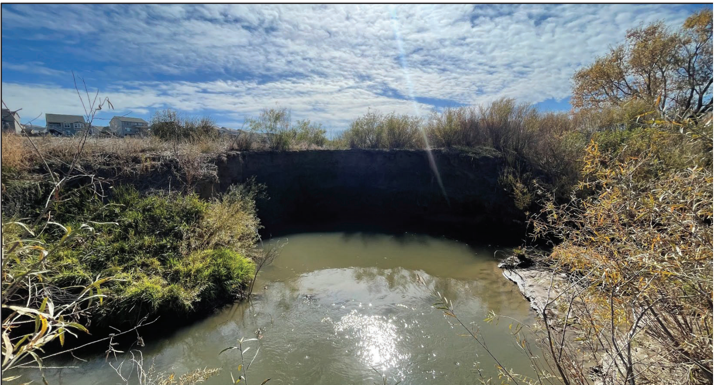
Severe incision has led to a lowered water table along the Little Thompson. Over time, this will cause stress to the riparian canopy. (10/25/24).
