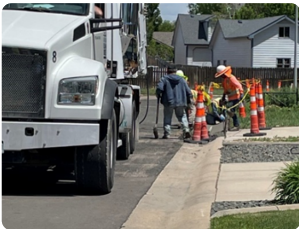
*Workers installing concrete in the street next to orange cones and a white truck.
