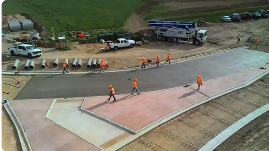
*Pavement placement east leg of roundabout construction
