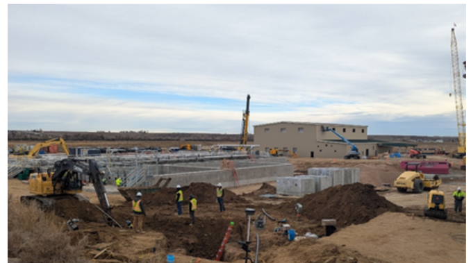
*Progress on the MBR Building
