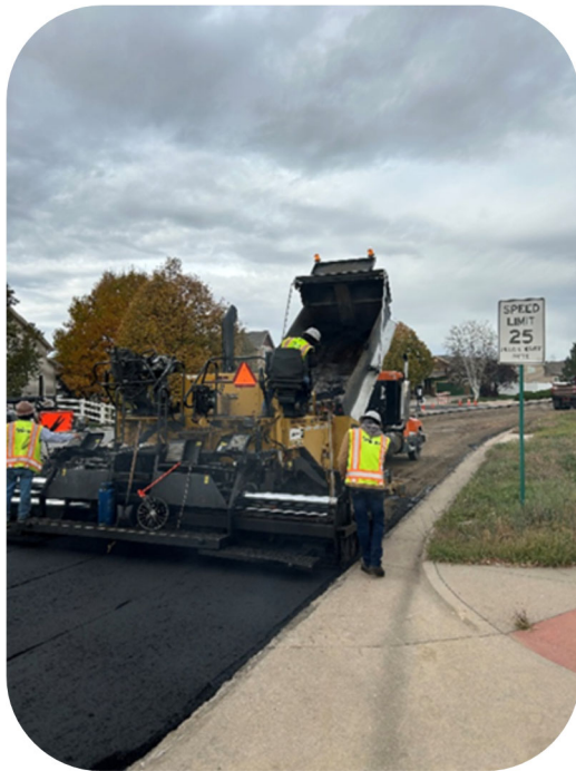
*Carlson Boulevard Paving
