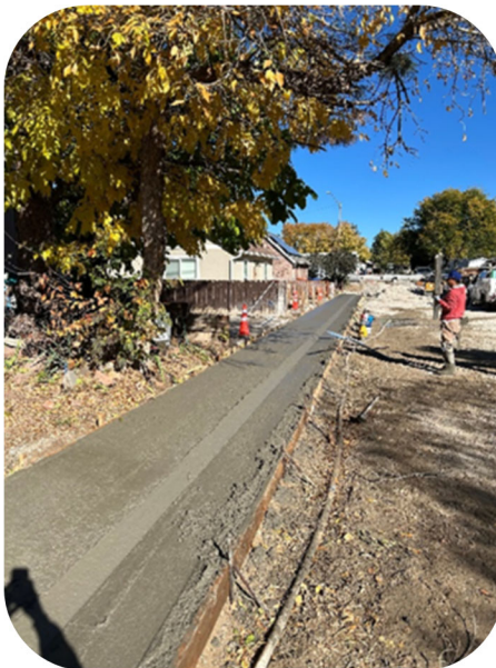
*New Curb, Gutter, and Sidewalk
