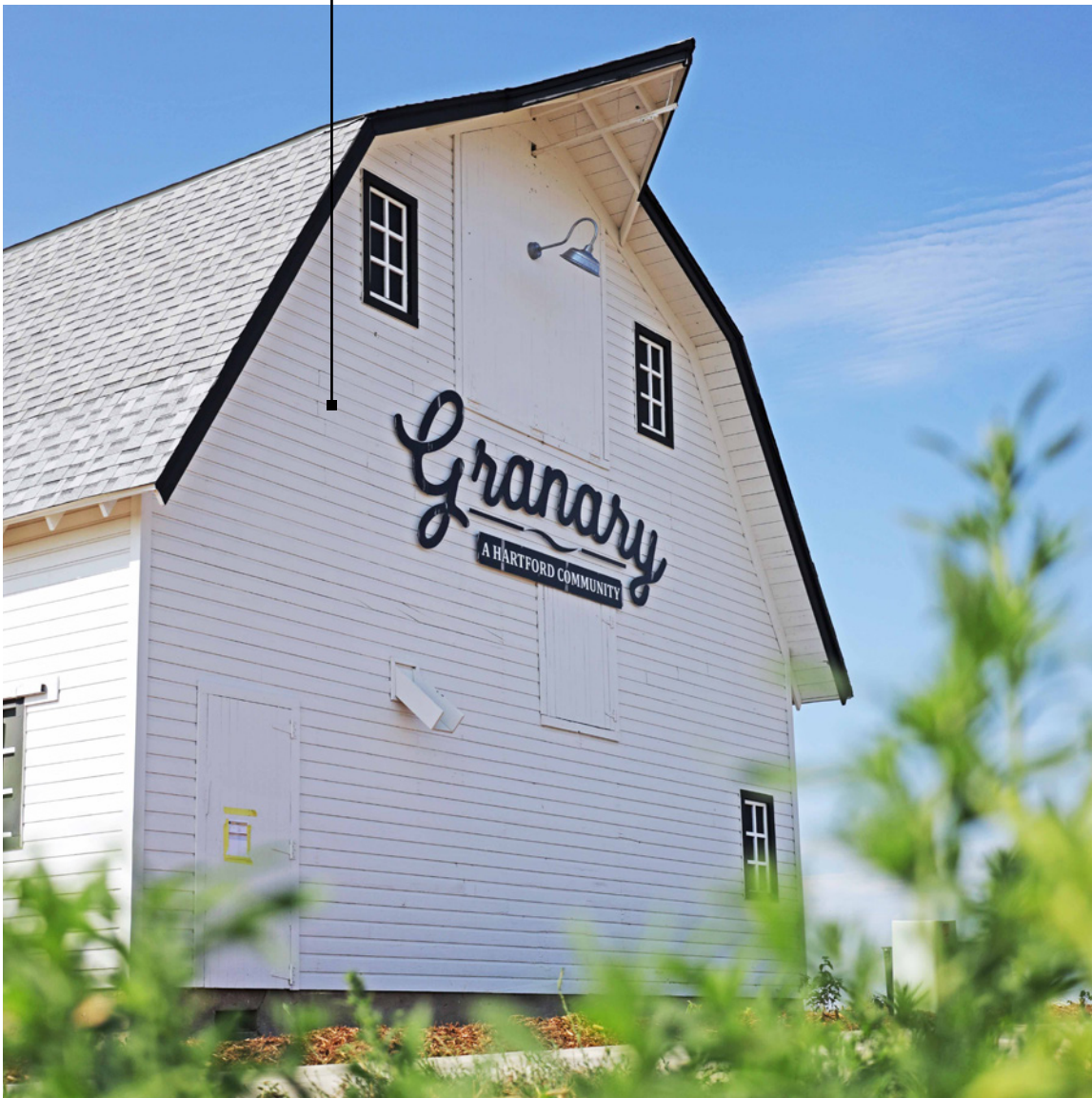
Reconstructed barn along Telap Avenue
