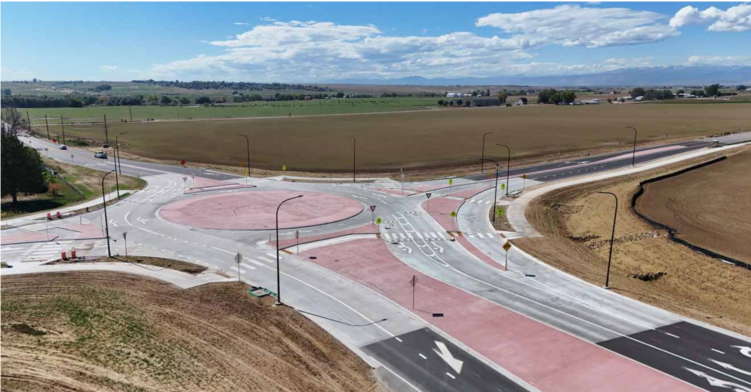
Roundabout (at west entrance along Colorado Blvd)
