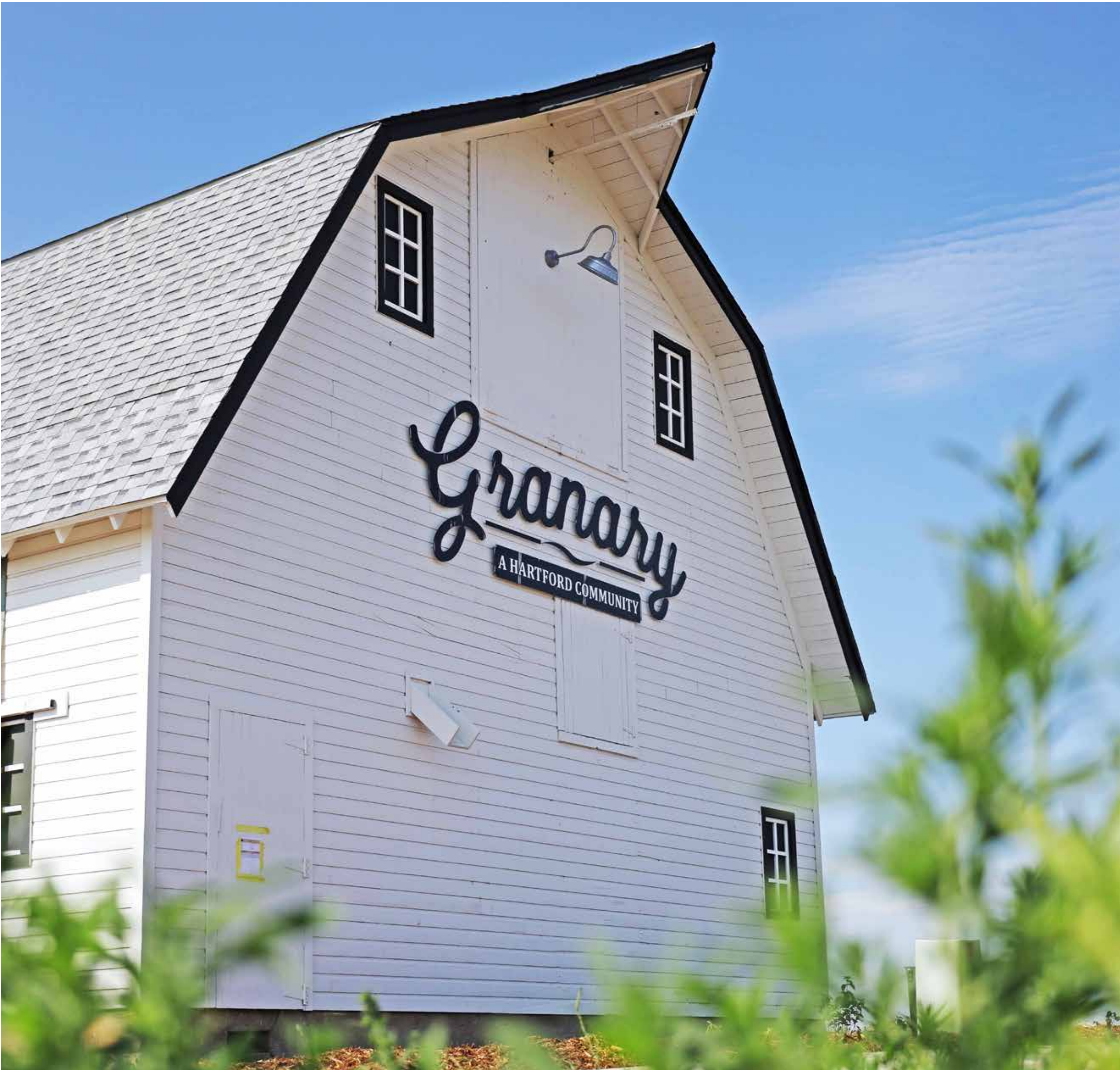
Restored Granary Entrance Barn (at east entrance along Telep)
