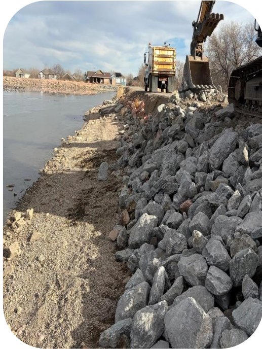
*Rip rap installation along the Johnstown Lake
