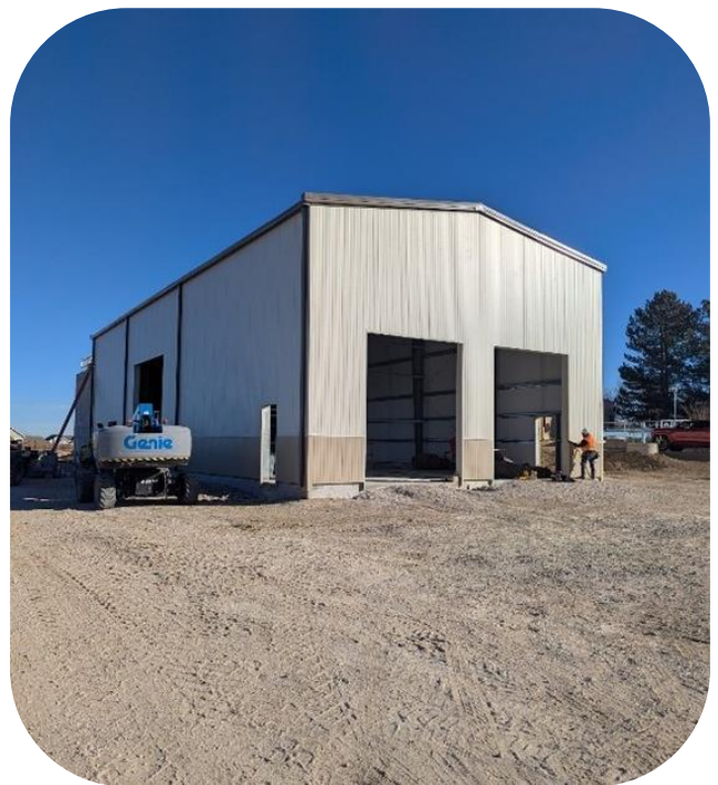
*Solids Handling Building
