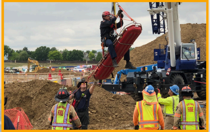
CONFINED SPACE RESCUE
