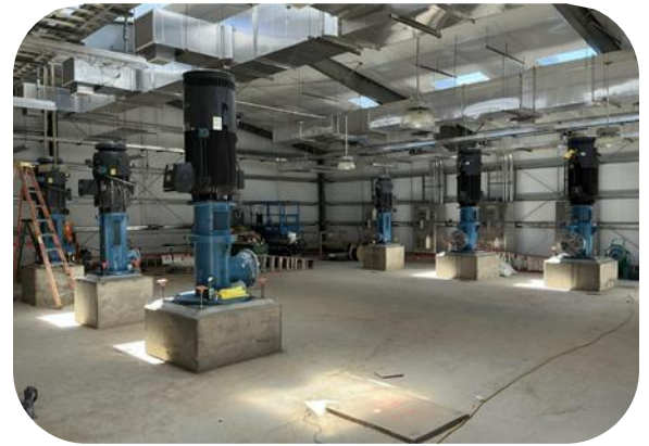
Final Vertical Turbine Pump Installation
