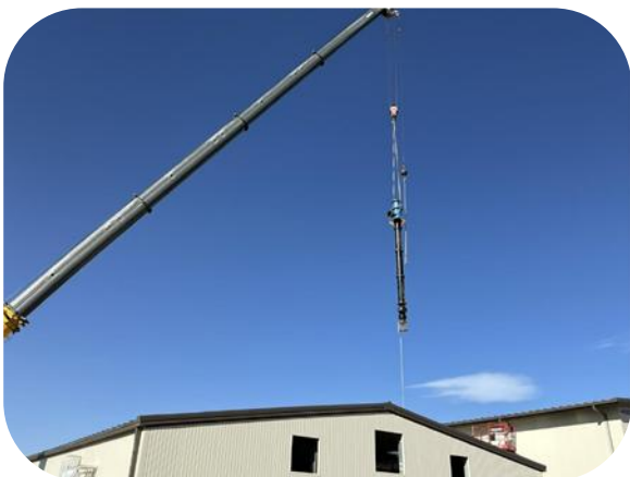
Vertical Turbine Pump Installation
